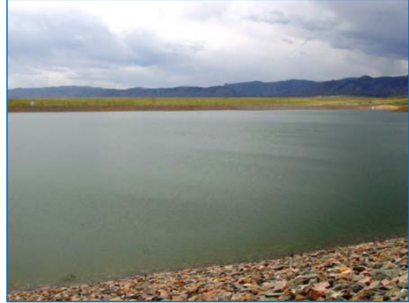
South Platte Reservoir has the capacity to store 6,400 acre feet of surface water for use by Centennial Water's customers in Highlands Ranch. The reservoir is approximately half full as of early May.
